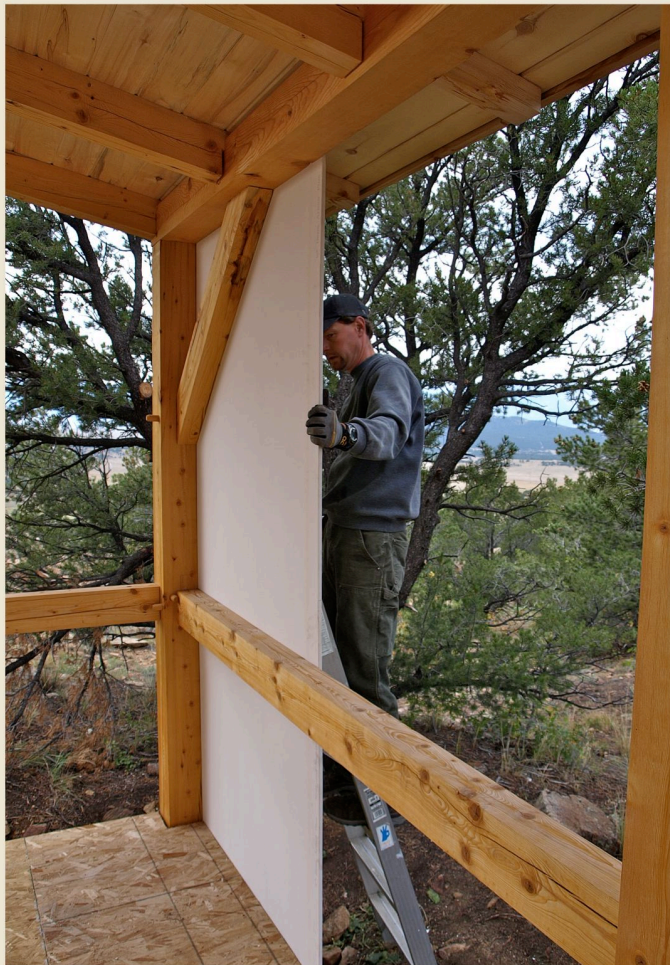
Kevin (left) screws a wall panel in place as closing-in begins. Pine siding (top) awaits installation. Cutout is ready for a picture window.
