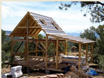
Aspen tongue-and-groove roof decking (top) has a fiery grain. Roofing goes on in stages.
