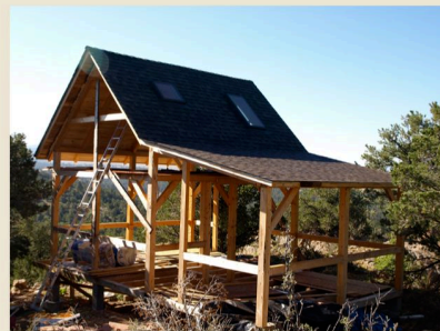
Aspen tongue-and-groove roof decking (top) has a fiery grain. Roofing goes on in stages.
