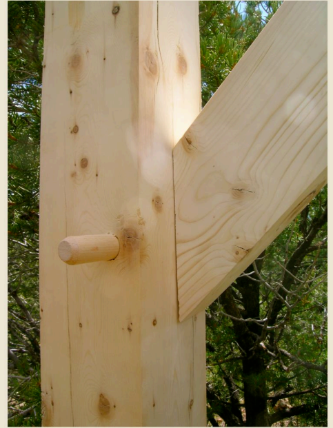
Facing page: Flooring timbers in place with first bent ready to be raised. | Above: First bent is braced into place. Detail of a brace joint.
