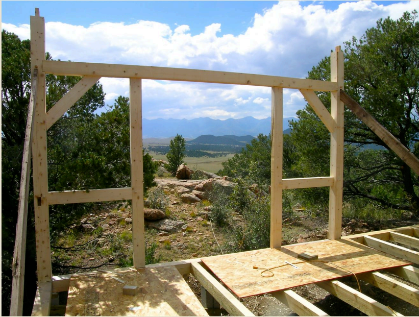
Facing page: Flooring timbers in place with first bent ready to be raised. | Above: First bent is braced into place. Detail of a brace joint.
