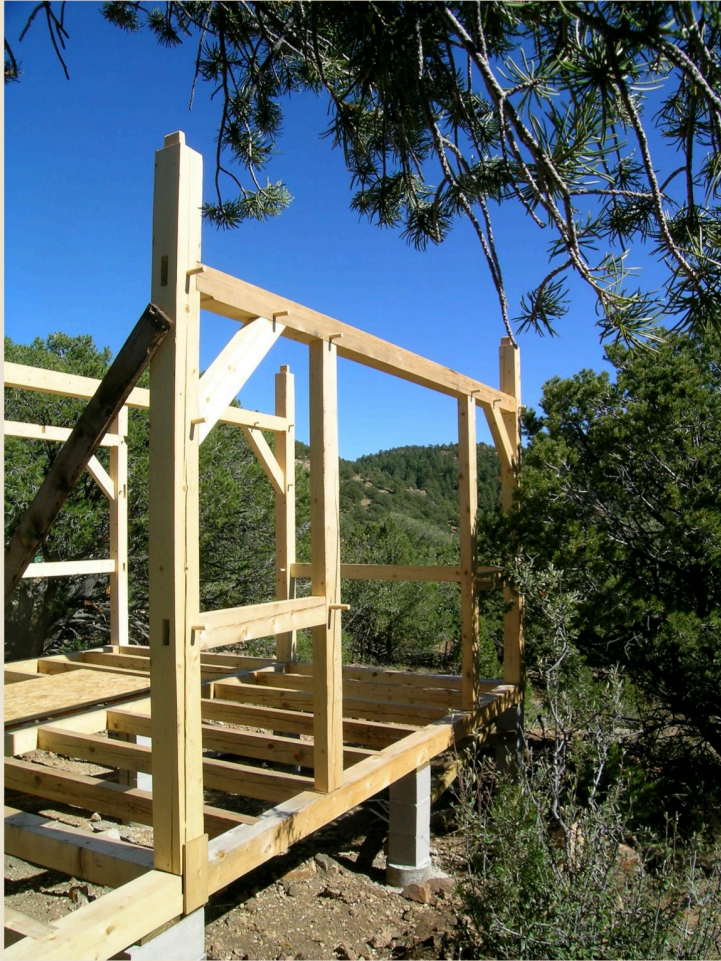
Above: The frame stands ready for top plate beams. Rafters await installation. | Facing page: Complex corner joinery in detail.
