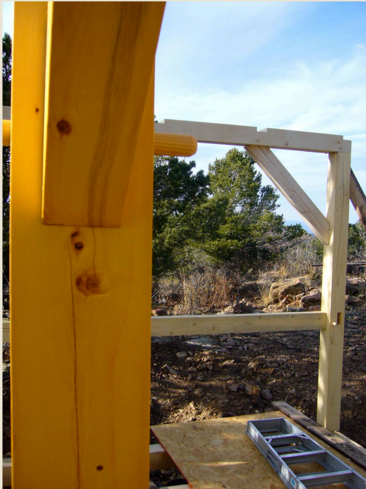
A post turns golden after being treated with a boiled-linseed/tung-oil mixture.
