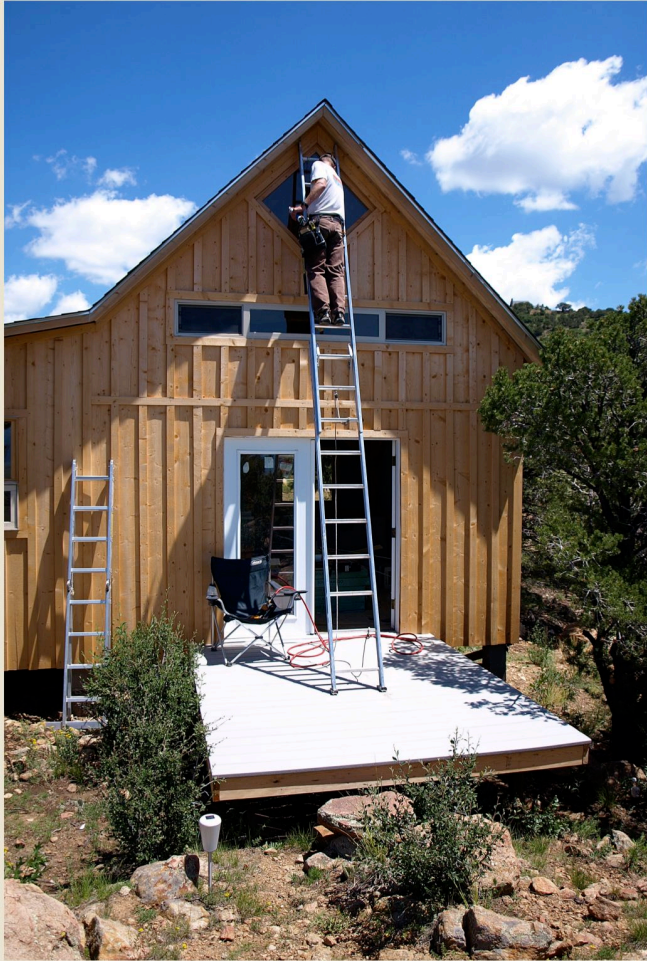
Kevin caulks the diamond-shaped window. Deck now in place. Bathroom walls (right) begin to go up in the area beneath the loft.
