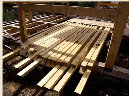
Above: The frame stands ready for top plate beams. Rafters await installation. | Facing page: Complex corner joinery in detail.
