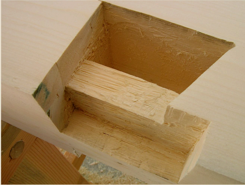
Left: A dovetail loft joist mortise after being cut into one of the posts. | Right: The author poses for a photo after raising the main frame.
